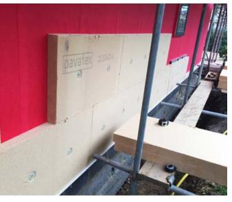
Breathable external insulation skin removes thermal bridges
