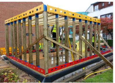
Factory cut steel easily combined with timber studs sourced through local builders merchants
