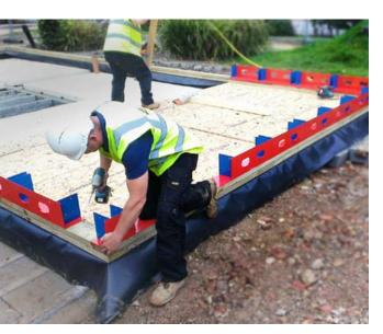
Self-adhesive airtightness and weather proof membrane bonded to OSB board and then fixed to timber studs
