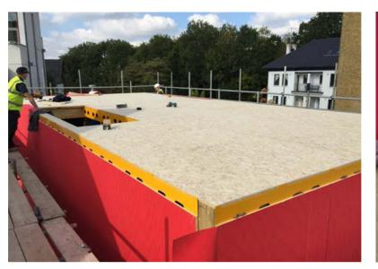
OSB fixed to floor joists
